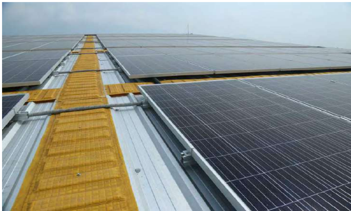
Jubilee Block at YIMS has 60 kW of SPV The energy is fed to the KSEBL grid and YIMS draws power from its existing connections
