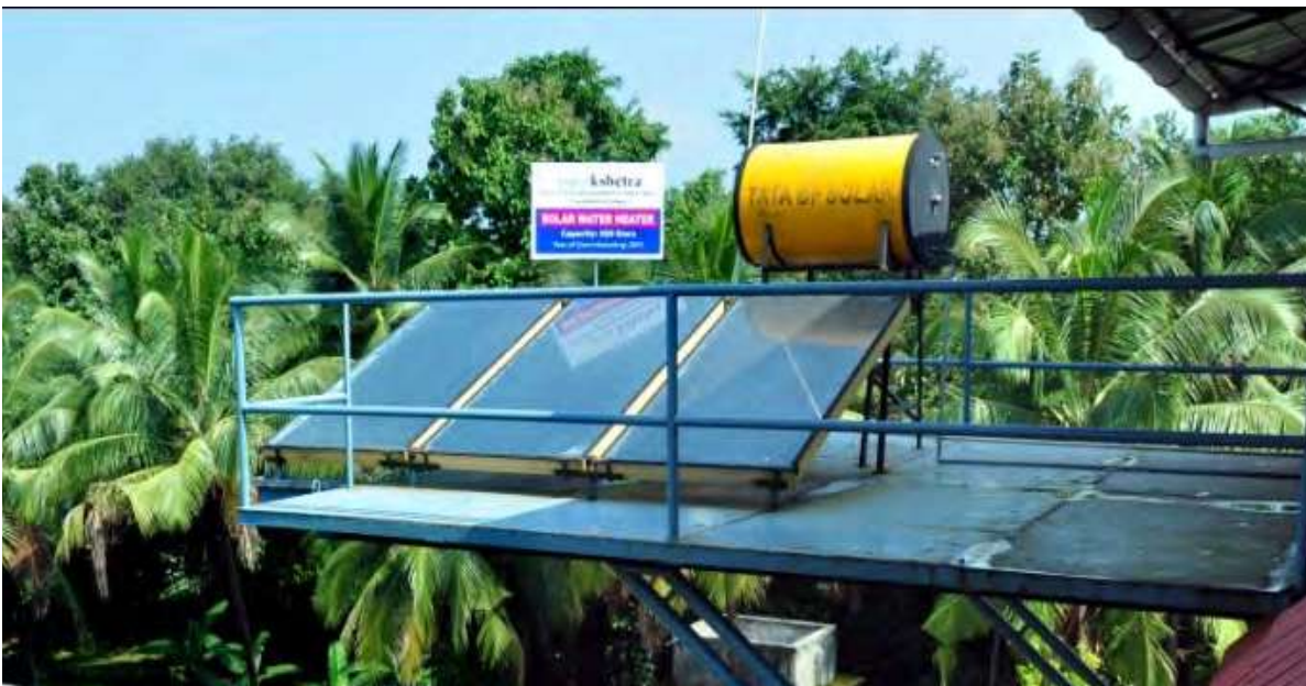
Solar Thermal Water Heating Systems (3 x 100 LPD) capable of raising water to 85°C Addition of Steam Cooker in hostel kitchen saves lot of fuelwood
